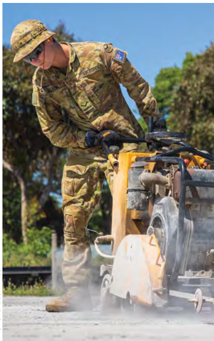
↑ A RAAF plant operator makes a cut in a concrete pad during airfield damage repair training at Basa Airfield during Exercise Balikatan, Philippines.
